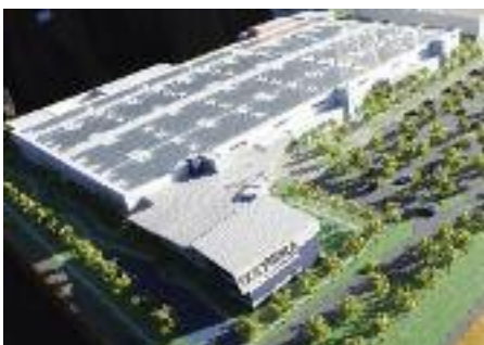
First phase of construction at Solyndra plant, a Local 595 project, will be a 600,000 square-foot photovoltaic manufacturing facility.
